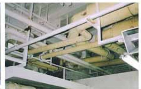
配管及防熱 Piping and insulation work
