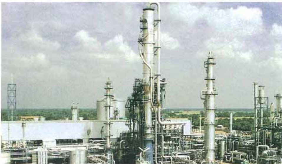
JF project OWNER Jamuna Fertilizer Co., Ltd. CONSTRUCTOR Mitsubishi Heavy Industries, Ltd. LOCATION Bangladesh
