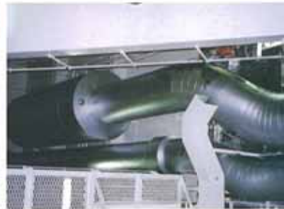
排ガス管防熱 Heat insulation of exhaust gas piping
