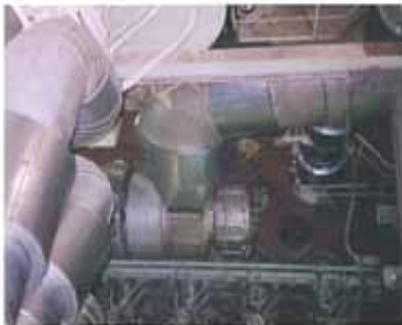
排ガス管防熱 Heat insulation of exhaust gas piping
