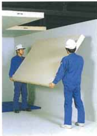
プレハブ冷蔵庫組立 Construction of Pre-fab ref. prov. chamber
